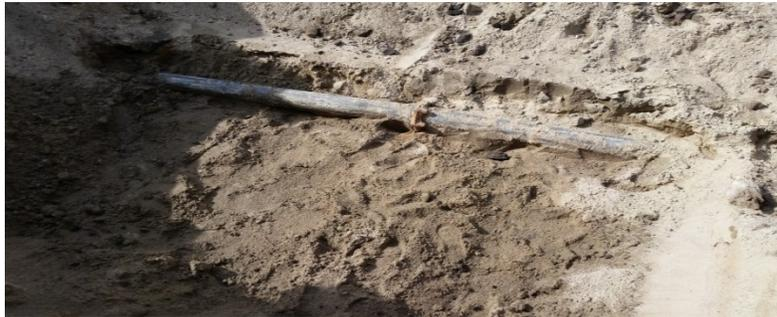
After recharging the water-line on July 23rd, a second break occurred approximately 2 miles further down the line towards town. The second break also occurred at the site of a repair made in the early 90's. A repair clamp was found less than a foot from a hole in the pipe repaired on July 26th. The sample of pipeline taken from this dig shows how the soil conditions have wreaked havoc on the original steel cast line put in during 1937-38.
